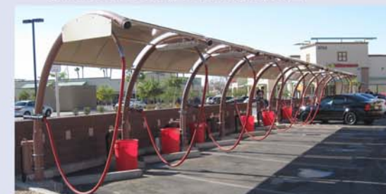
Arch Stanchion with Steel Awnings, Quick N Clean, Glendale, AZ
