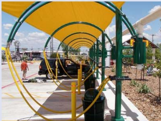
Arch Stanchion for Overhead Pipe Car Wash Barn, Killeen, TX
