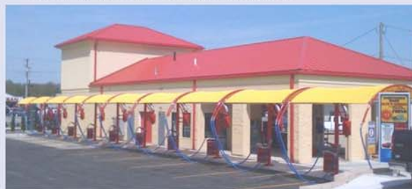
Arch Stanchion, Overhead Piping, Speed Wash, Somerset, KY
